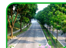
Well- Laid Bitumen Roads
